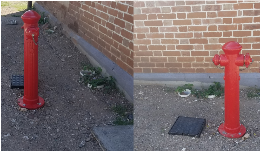
New Fire Hydrants
