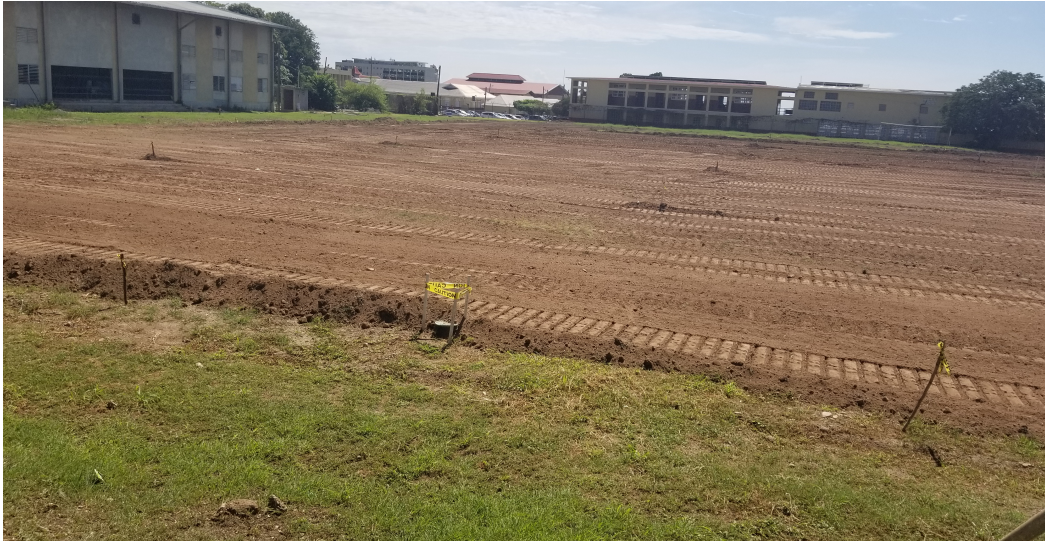
Cutting and levelling of the Football Field
