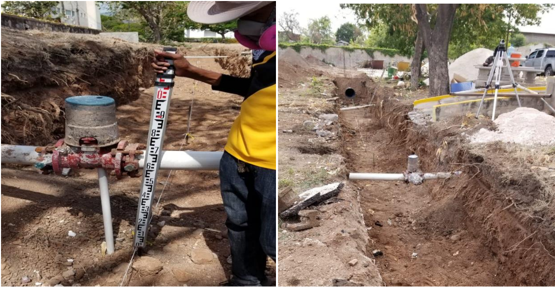
Construction of the drainage system
